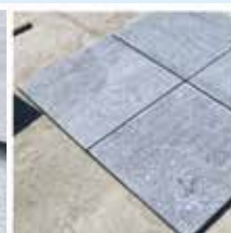
INSTALLATION ON CEMENT
