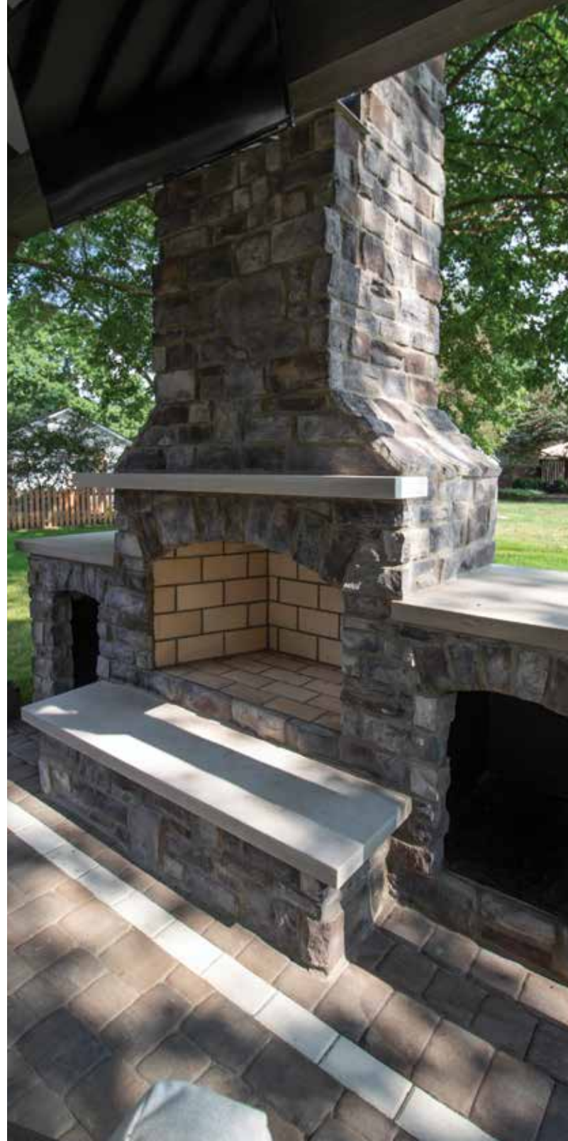
Round Grove Fireplace and Two Wood Boxes finished with ProVia Terra Cut Slate
