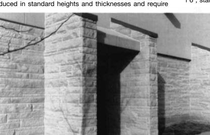
no additional work other than cutting to proper length on the job. Ashlar veneer and its matching trim are set in mortar like any unit masonry product, and may be applied to any type of backup as illustrated in the two following pages. With ashlar veneer, no shop drawings or anchors are included, and the stone is priced per ton.
